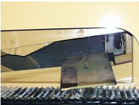
10:- Lower existing toggle onto main conveyor. - remove & replace with new toggle plate.
