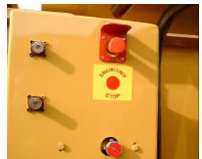
3:- Emergency stop on L/H side of crusher box.
