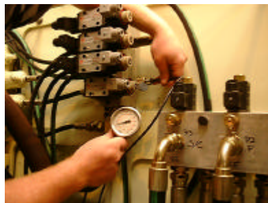
Check control pressure using a 0 - 100 bar pressure gauge. This should be 40 bar at all times.
