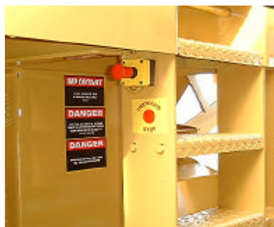
2:- Emergency stop on L/H walkway ladder.
