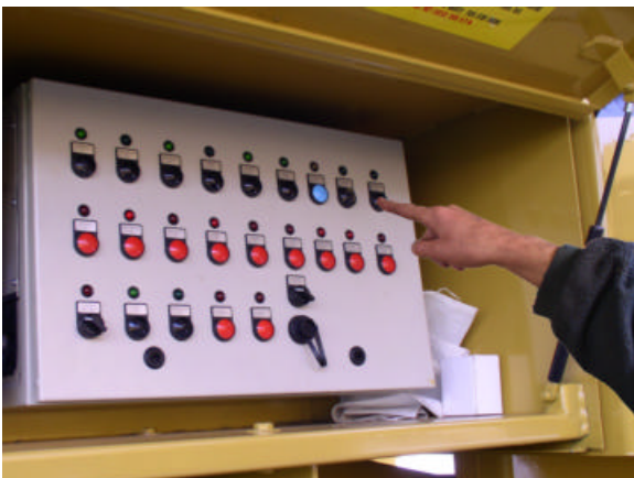
3:- Press button "Main conveyor lift"
