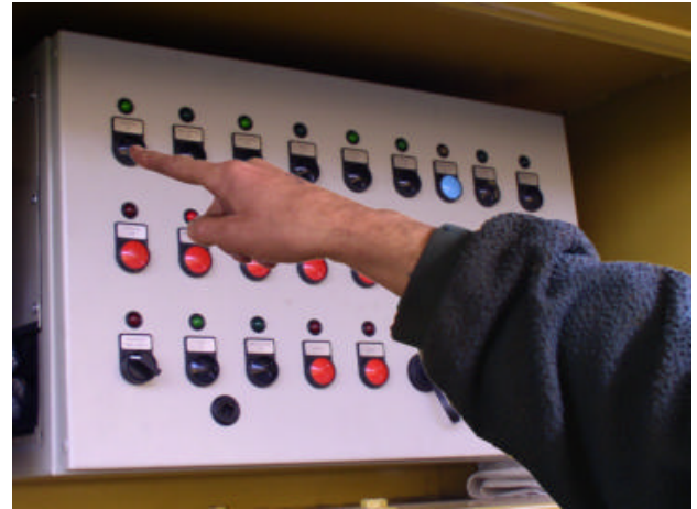
2:- Press button "Interlock On"
