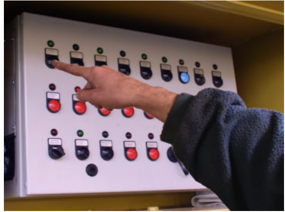
2:- Press button "Interlock On"
