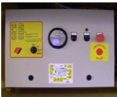
1:- Emergency stop & ignition switch in control box.
