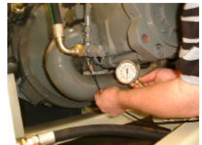
Check suction pressure using a 0 - 6 bar pressure gauge - this should be 1/2 bar min. - 1 1/2 bar max.
