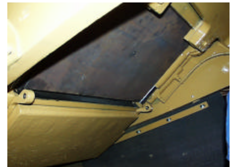
12:- Raise new toggle plate into position.
